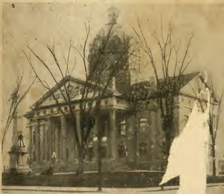
BROOME COUNTY COURT HOUSE, BINGHAMTON, NEW YORK
